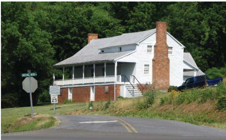
Intersection of SR 126 and Chestnut Ridge Road
