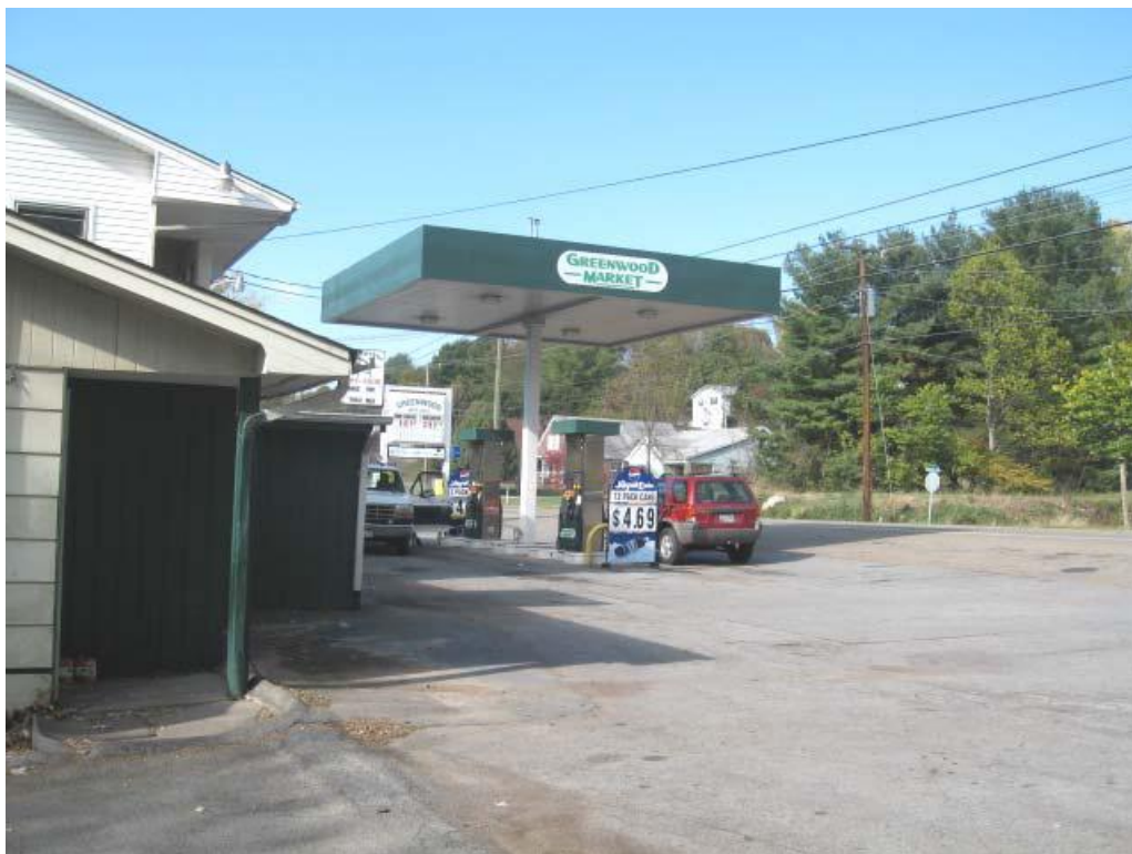
FIGURE 4.16.4: MARKET AND DELI AT 5121 MEMORIAL BOULEVARD
