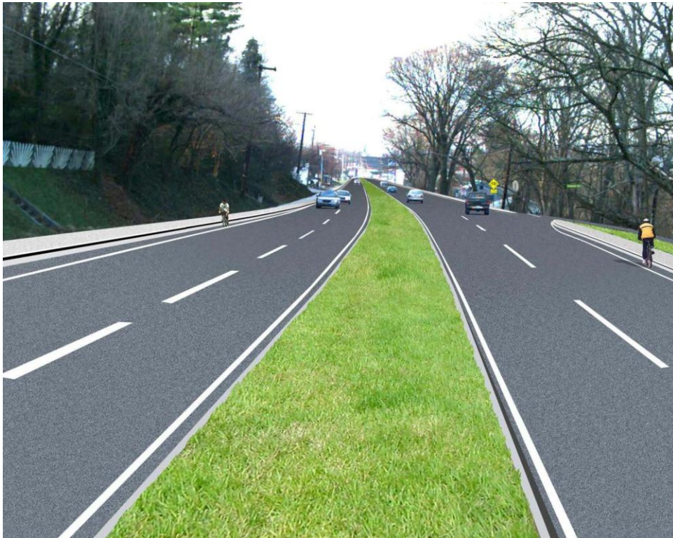
FIGURE 2.3.11: SEGMENT 3A PROPOSED TYPICAL SECTION 4-Lane, Raised Median, Shoulders, Curb & Gutter, & Sidewalks
