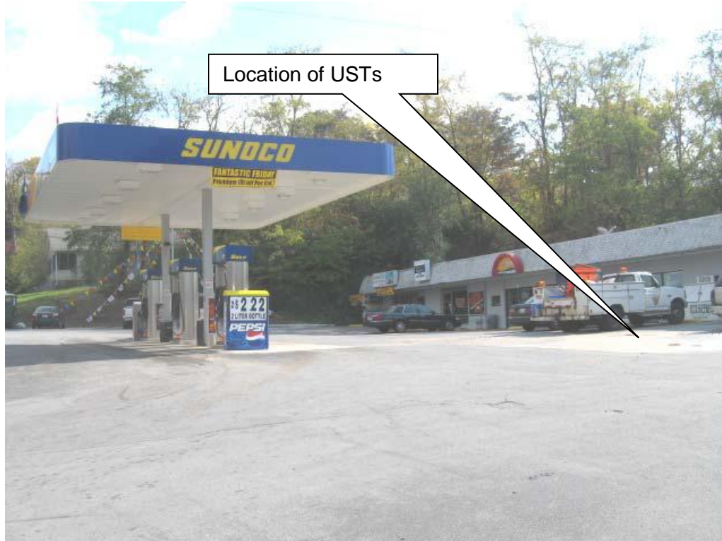
FIGURE 4.16.2: GAS STATION AT 4001 MEMORIAL BOULEVARD
