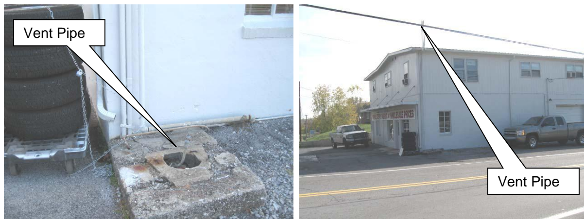
FIGURE 4.16.3: FORMER GAS STATION AT 5001 MEMORIAL BOULEVARD – EVIDENCE OF TANK REMOVAL
