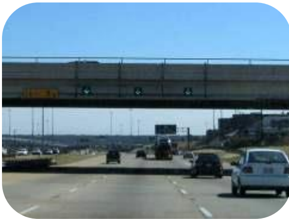
Lane Control Systems
