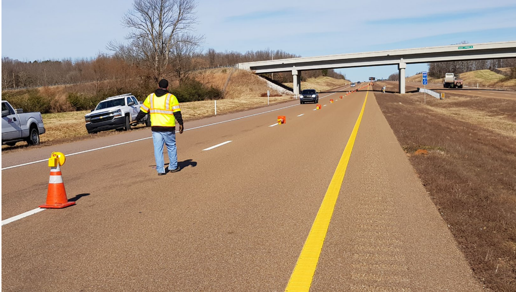
Figure 4-28. Project 2: Traffic cones knocked down by gusts from passing vehicles
