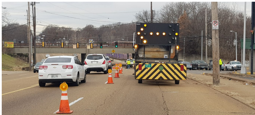
Figure 4-30. Project 3: LEDs on Intellicone sensors
