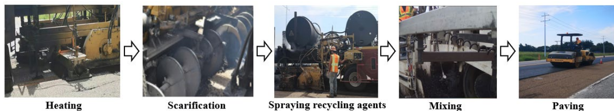
Figure 2-1. Hot in-place recycling procedures.
