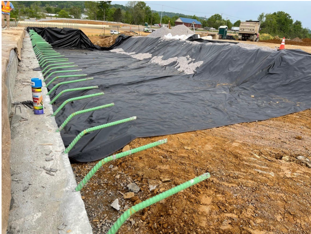
Figure 3-3. Propex GEOTEX-315ST Geotextile fabric laid at the bottom before placing the fill for the north approach slab.
