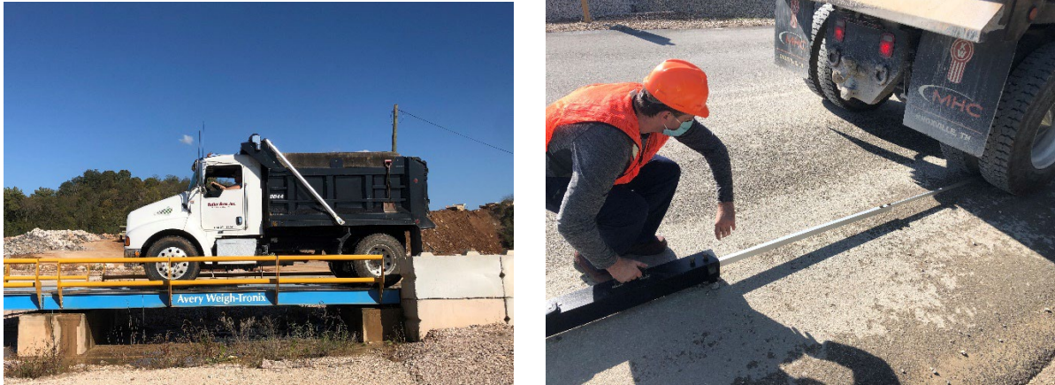
(a) (b) Figure 4-17. Overview of the Benkelman beam test
