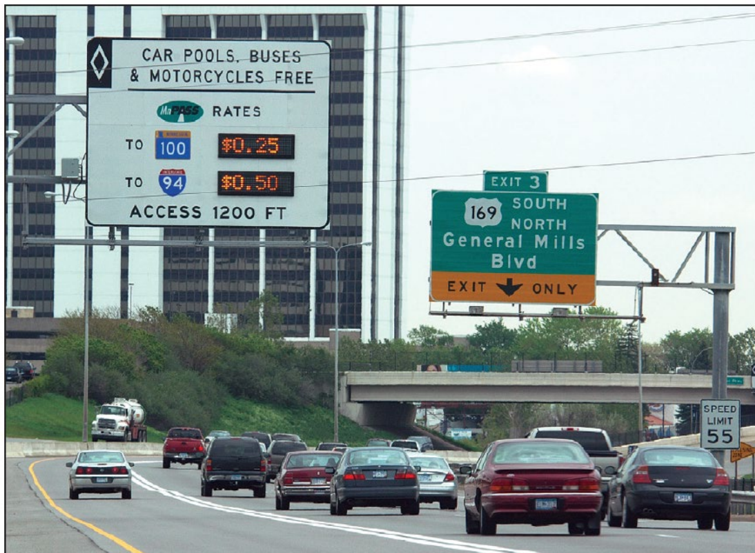
Figure 2.2: I-394 Pass in Minnesota (HOT Lanes)
