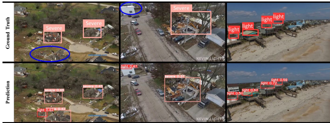
Figure 4-5 Visualization of Detected Damaged structures.
