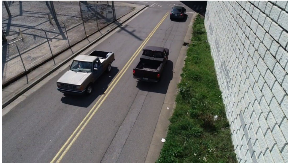
Figure A. 5 Fairly good vegetation at the foot, no soil erosion and deflection/displacement observed
