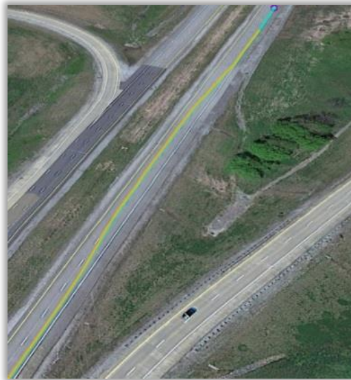
Figure 30 – Test Path – Following Accuracy on Lane Change Test
