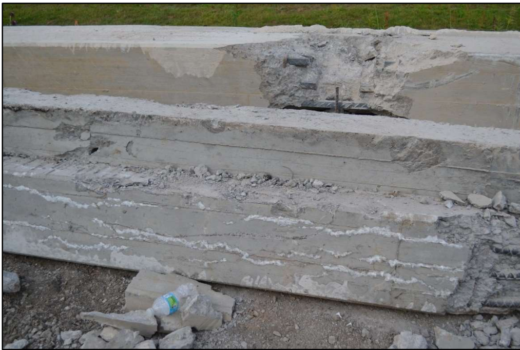
Figure 4-22: Superstructure - Deterioration
