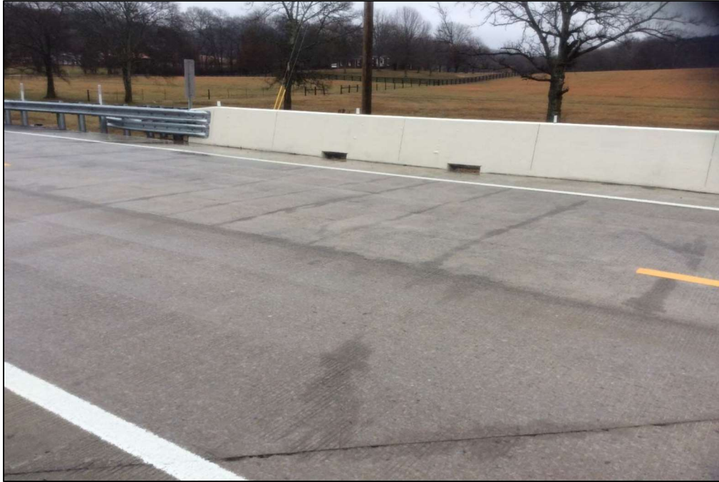
Figure 4-49: Completed Deck – Bridge No. 94-SR11-0.59
