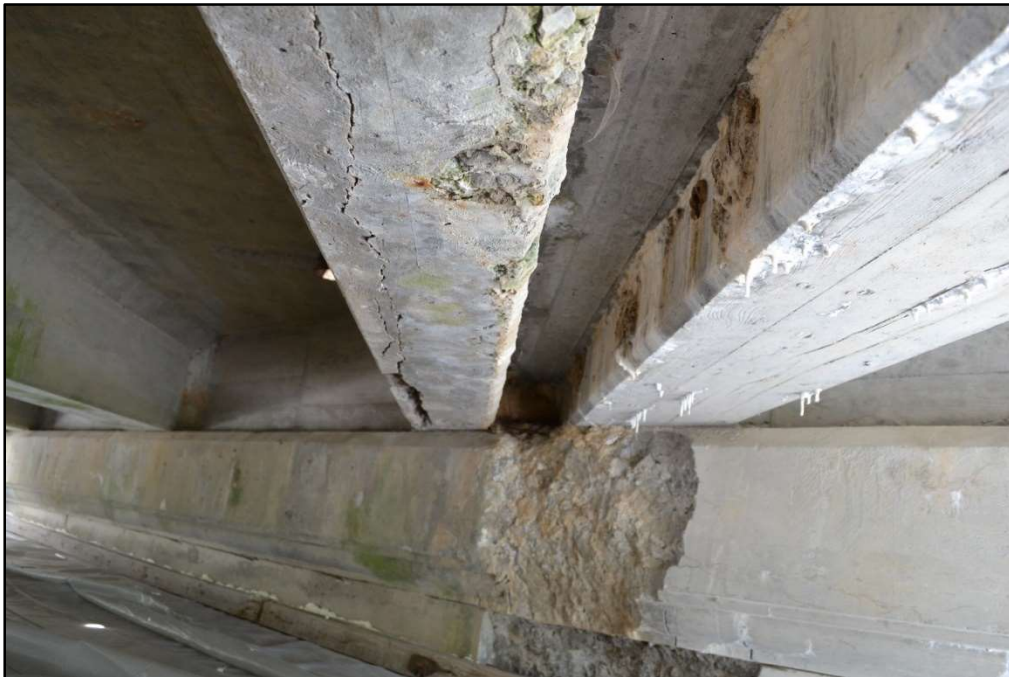
Figure 4-18: Superstructure - Deterioration
