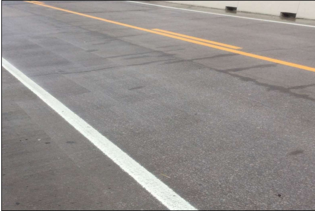
Figure 4-61: Completed Deck – Bridge No. 94-SR11-0.87
