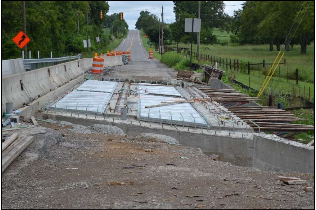
Figure 4-36: Deck – Form Installation
