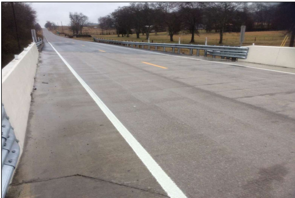
Figure 4-50: Completed Deck – Bridge No. 94-SR11-0.59
