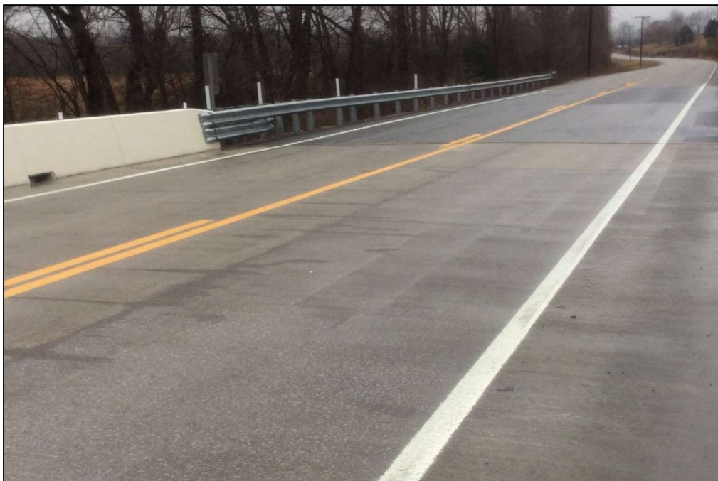
Figure 4-62: Completed Deck – Bridge No. 94-SR11-0.87
