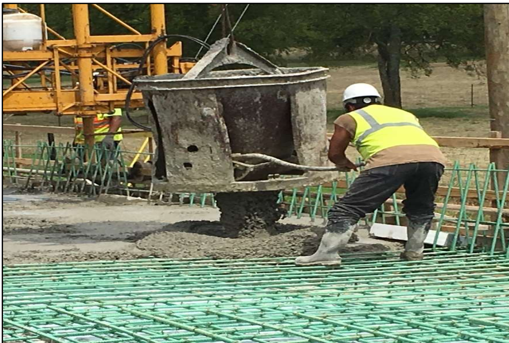
Figure 4-42: Deck – Concrete Placing
