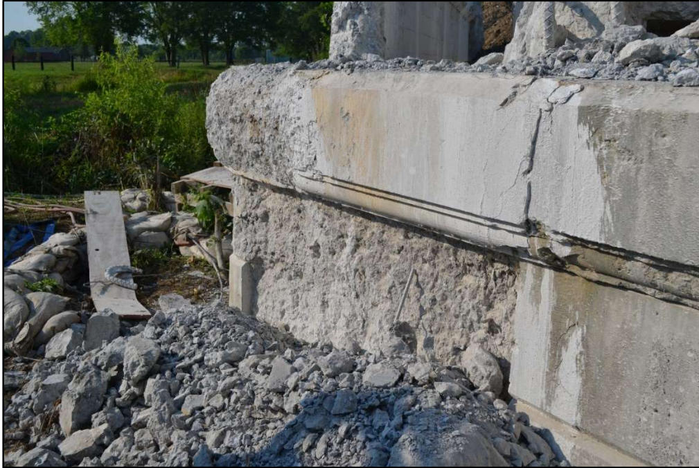
Figure 4-7: Substructure - Deterioration
