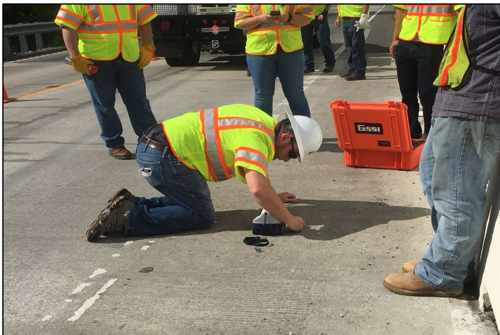
Figure 5-40: Locating Reinforcing Steel
