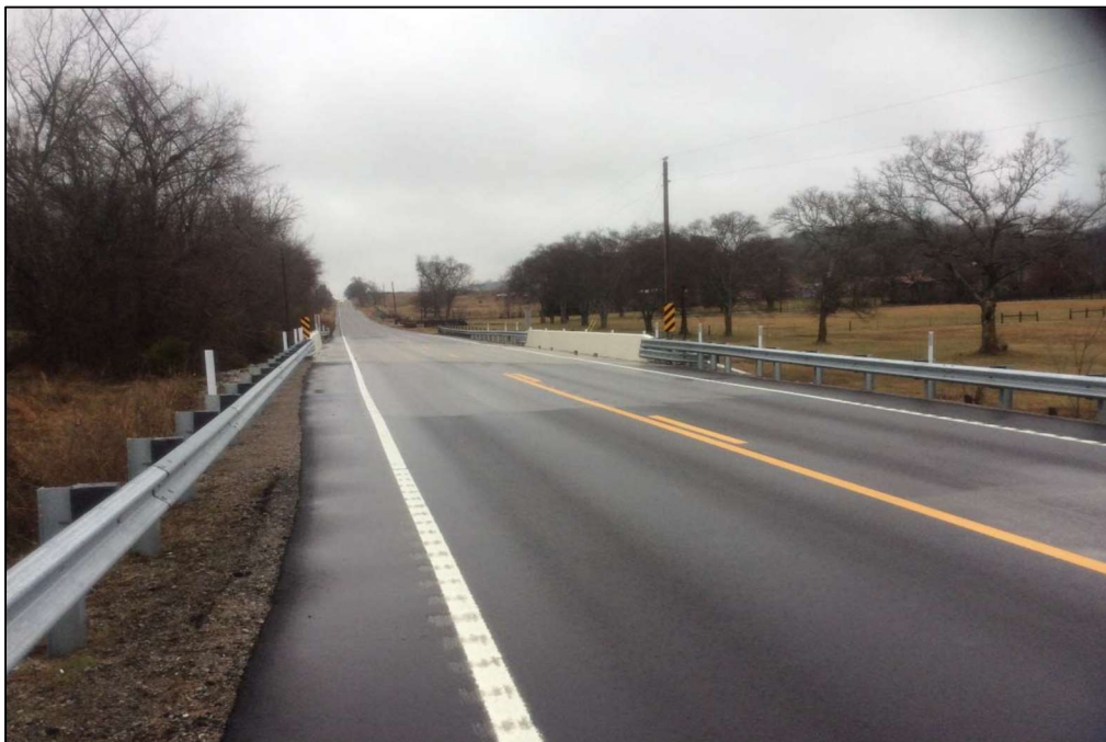
Figure 4-44: Completed Deck – Bridge No. 94-SR11-0.59
