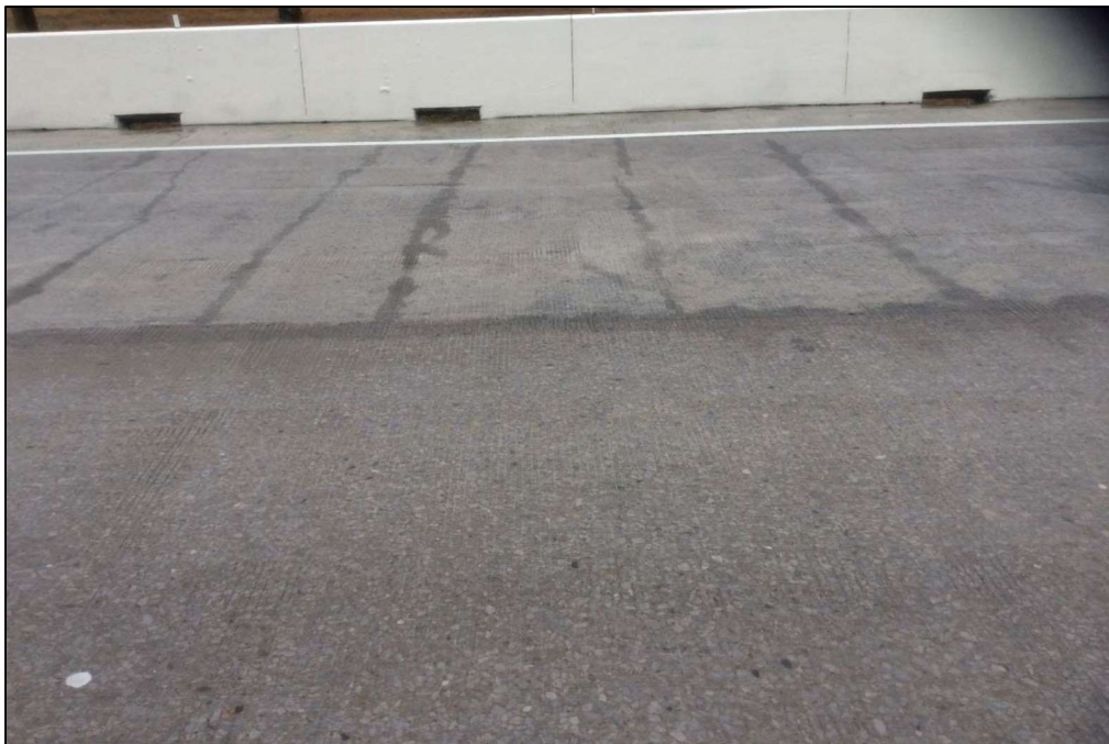
Figure 4-54: Completed Deck – Bridge No. 94-SR11-0.59
