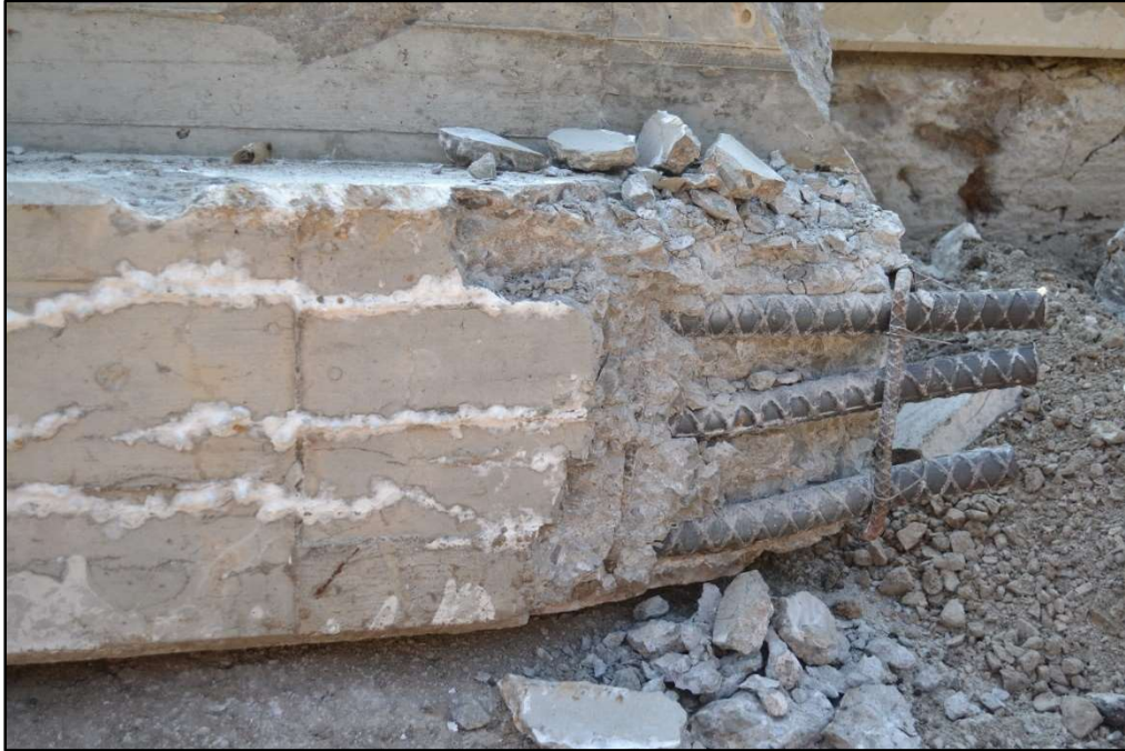
Figure 4-21: Superstructure - Deterioration
