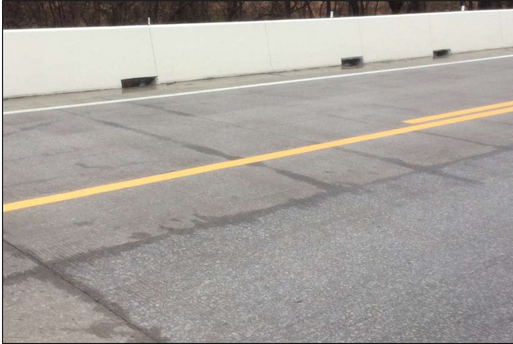
Figure 4-63: Completed Deck – Bridge No. 94-SR11-0.87
