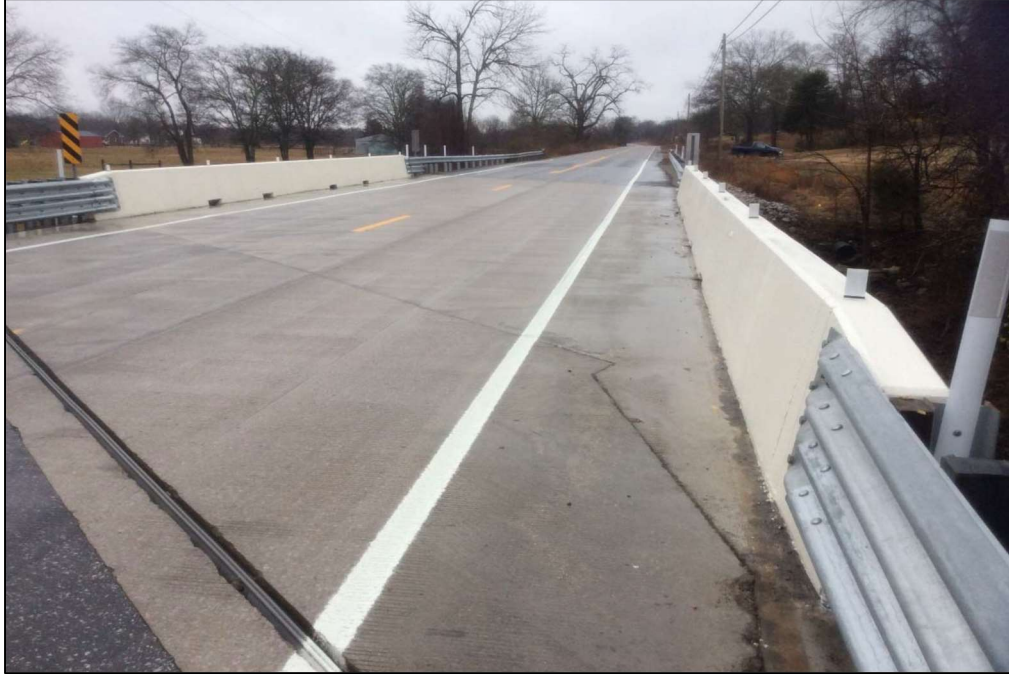
Figure 4-55: Completed Deck – Bridge No. 94-SR11-0.59
