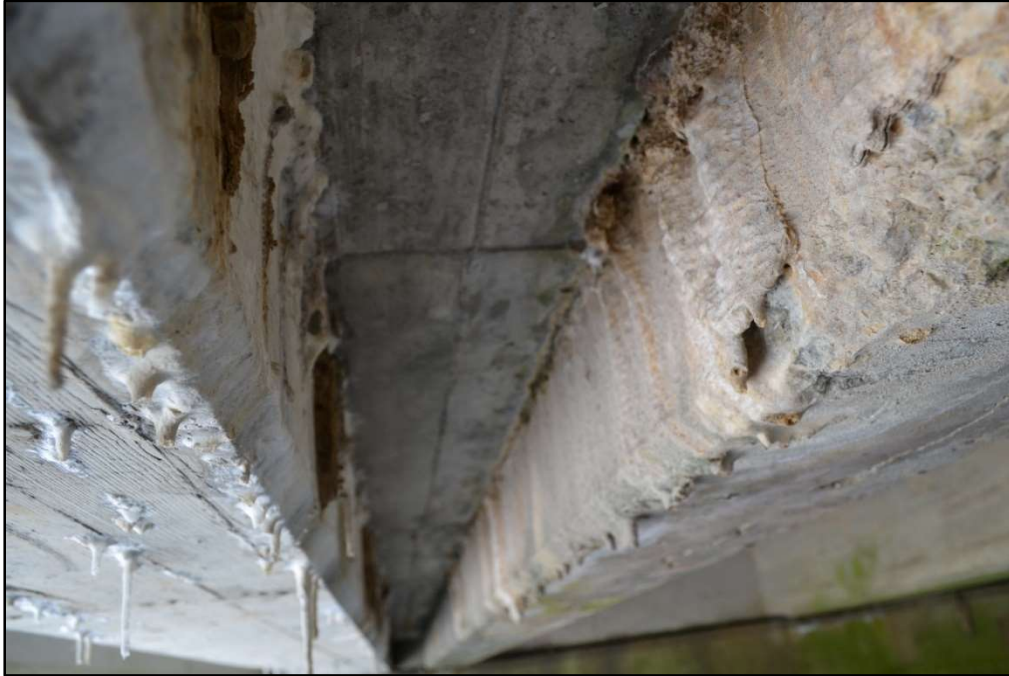
Figure 4-17: Superstructure - Deterioration
