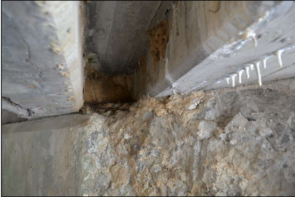
Figure 4-5: Substructure – Deterioration
