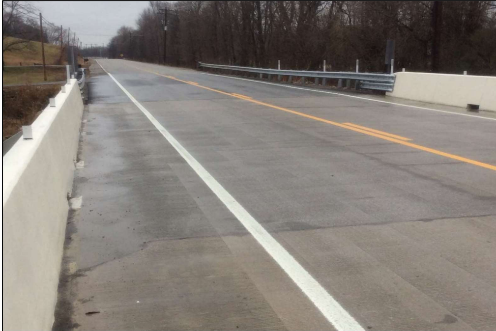
Figure 4-59: Completed Deck – Bridge No. 94-SR11-0.87
