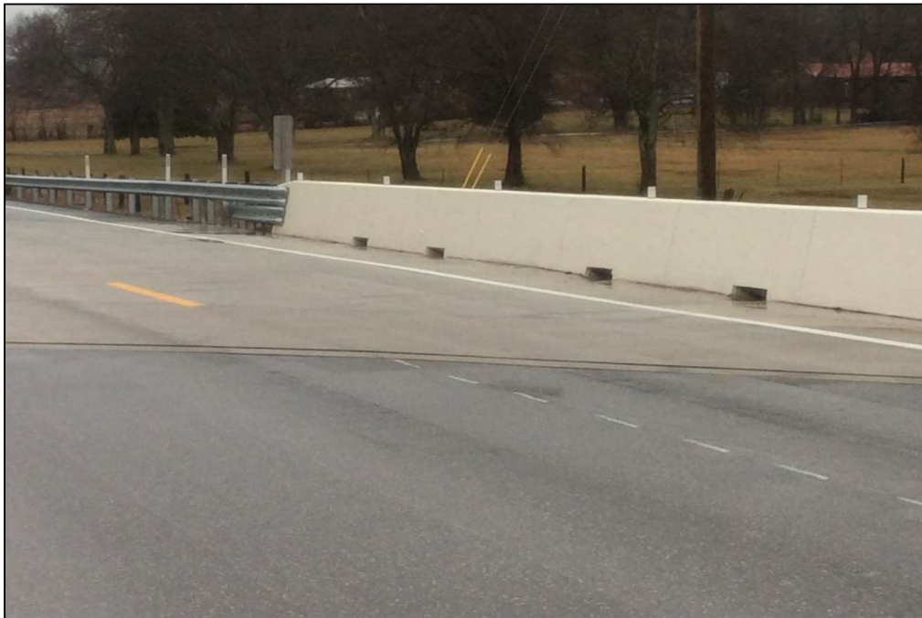
Figure 4-46: Completed Deck – Bridge No. 94-SR11-0.59
