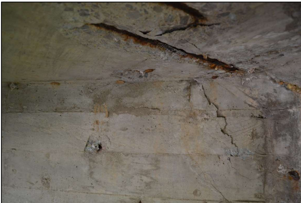
Figure 4-28: Deck - Deterioration
