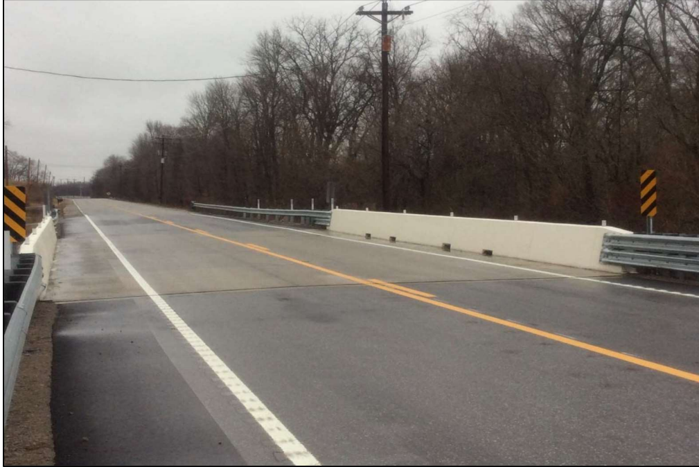
Figure 4-57: Completed Deck – Bridge No. 94-SR11-0.87
