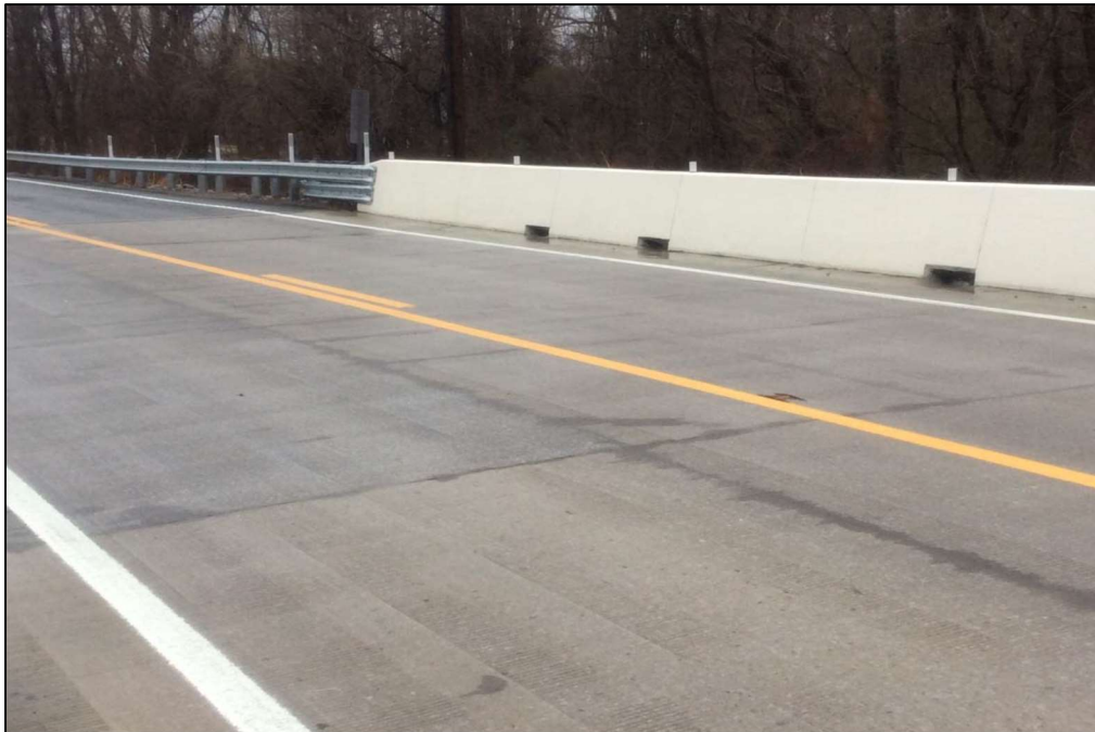
Figure 4-58: Completed Deck – Bridge No. 94-SR11-0.87
