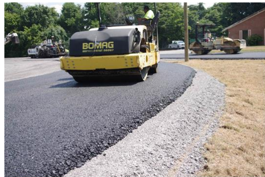
(a) Roller for soil compaction (b) Roller for asphalt mixture compaction
