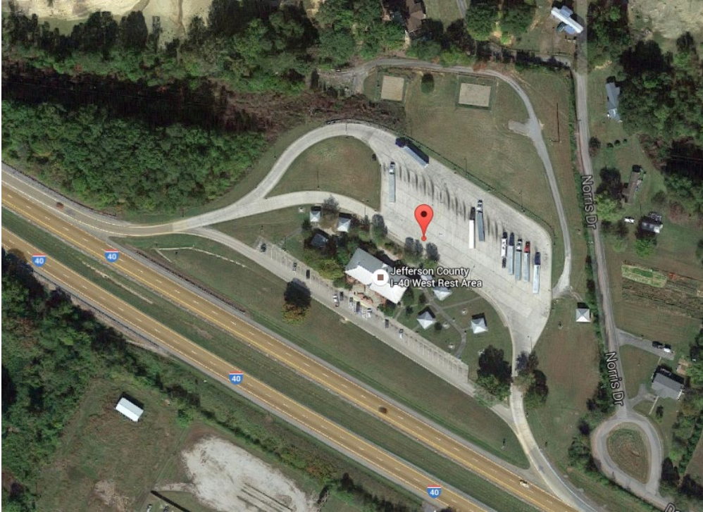
Figure 12: Rest area 41, Jefferson County I-40 West rest area
