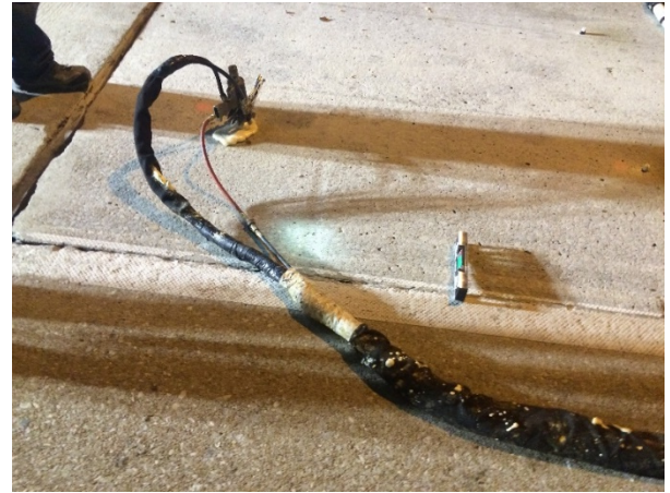
Figure 3.4 Drilling holes and installation of PolyLevel® materials on I-24 West
