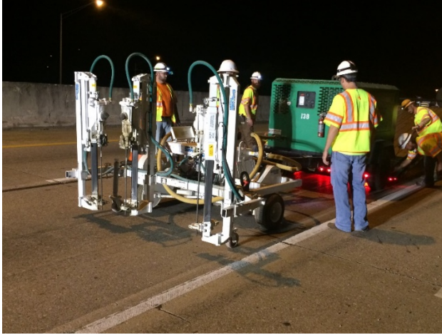
Figure 3.4 Drilling holes and installation of PolyLevel® materials on I-24 West
