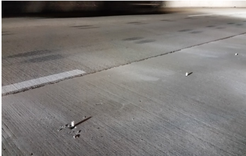
Figure 3.6 Injection holes on concrete slabs
