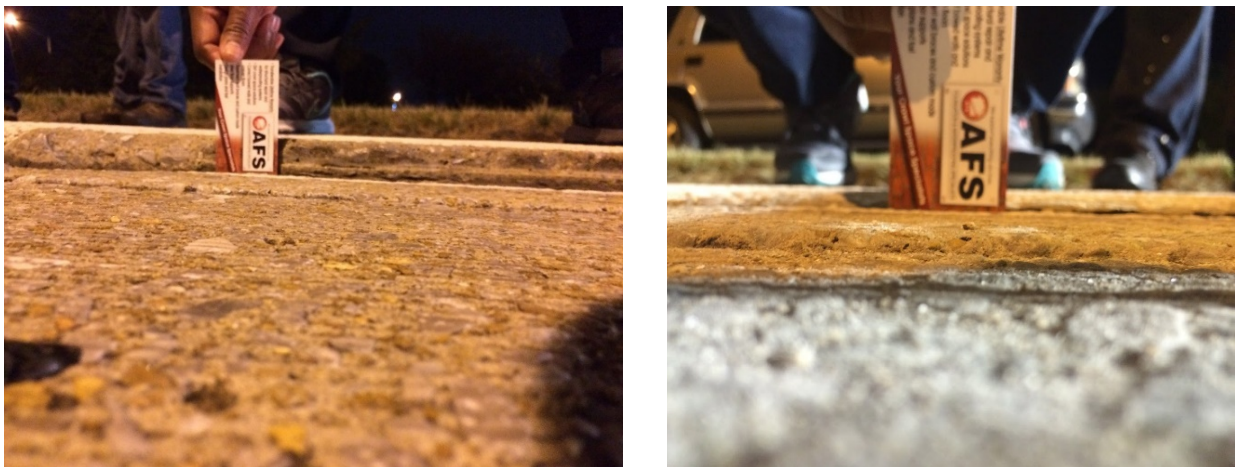
Figure 3.3 Before and after leveling slabs using PolyLevel® material on I-24 West
