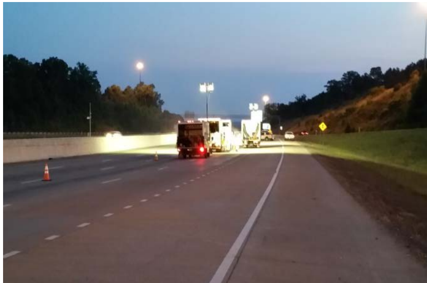
Figure 3.5 View of I-75 South
