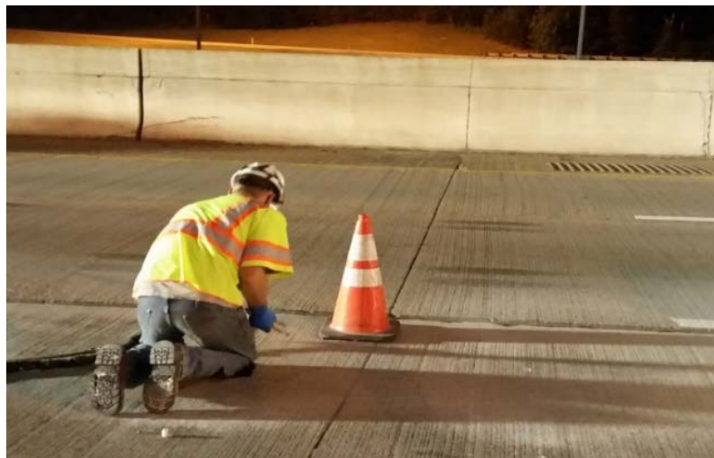
Figure 3.7 PolyLevel® injection on I-75 South
