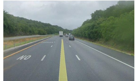
Figure 3. Left lane added for passing trucks on I-40 eastbound in Smith County
