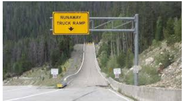
Figure 33. Runaway Truck Ramp (Colorado DOT)
