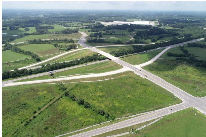
Figure 42. Recently constructed interchange at I-40 and Tennessee Avenue in Cookeville (HMB)
