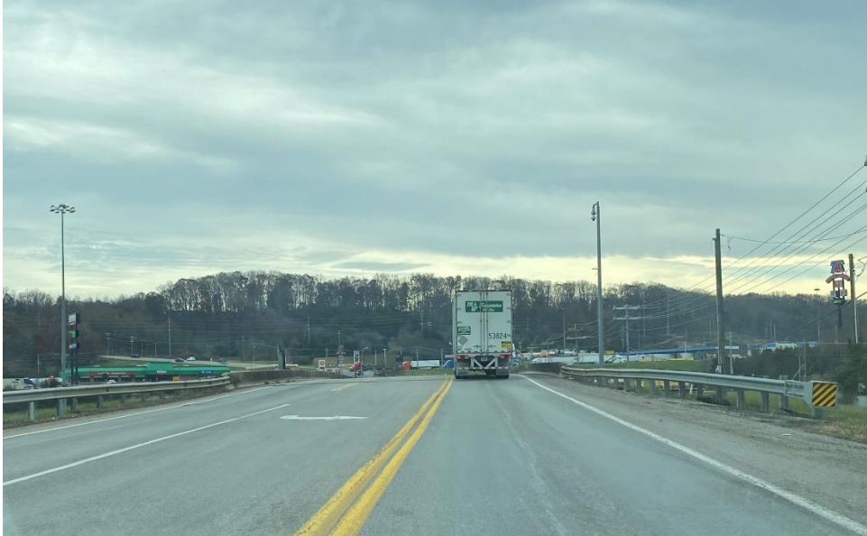
Figure 5. Watt Road Looking South – Approaching Existing Bridge
