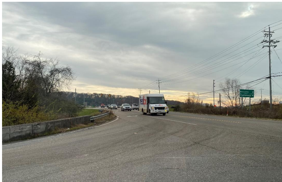
Figure 7. Looking South from Everett Road - Just North of Interchange
