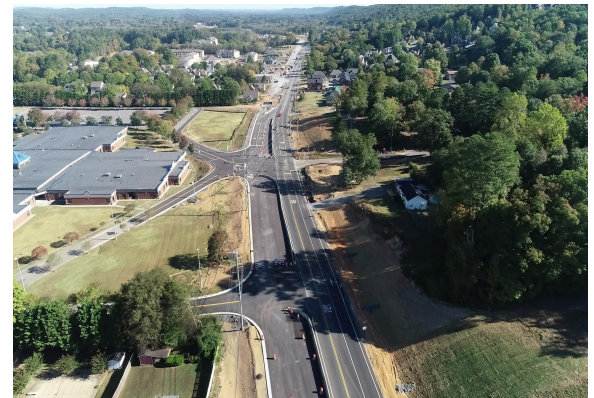
Widening near Cleveland Middle School
