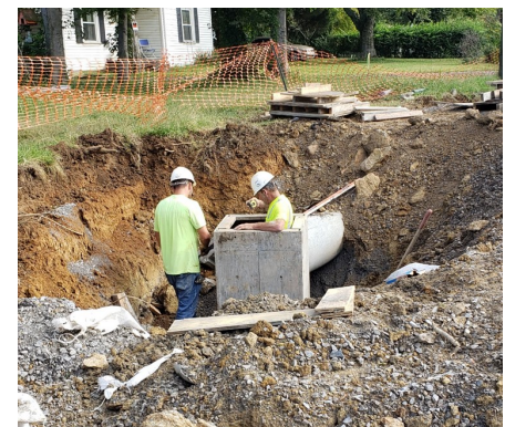
Subcontractor installing storm drain structures within Courtney Avenue.
