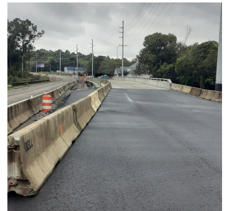
Bridge over Whites Creek
