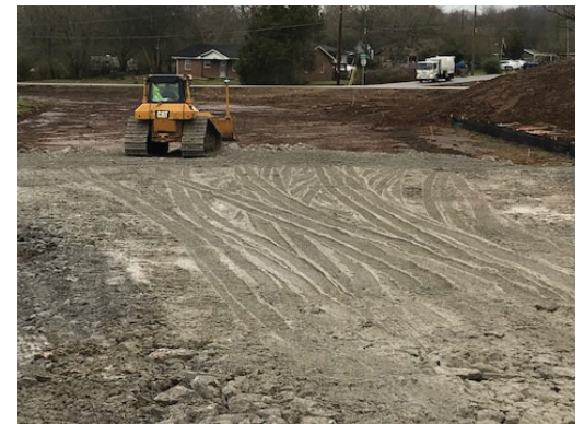
Grading work at new W. Hamilton Rd. alignment
