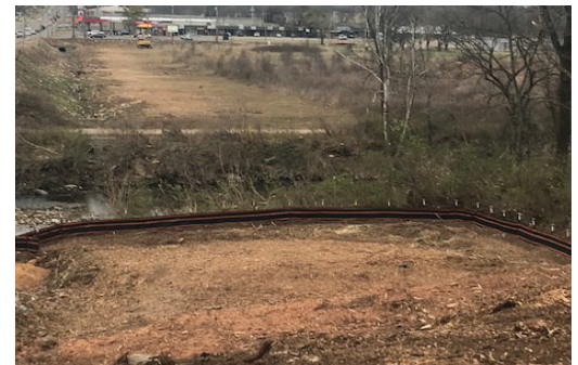
Clearing and installation of erosion measures
