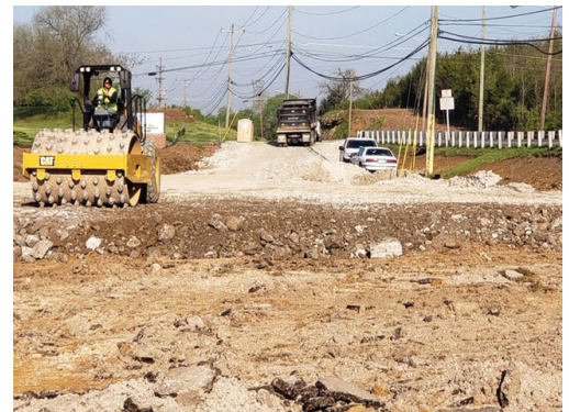
Placement of fill material for the roadway base near the YMCA.
