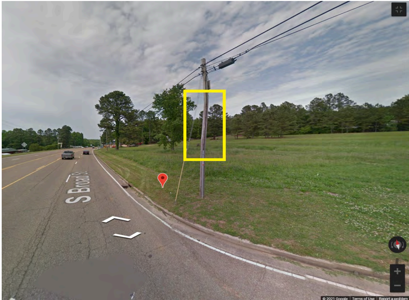
Camera 3, installed on existing wooden utility pole on Hwy 22 near Tignor Park Lane.
