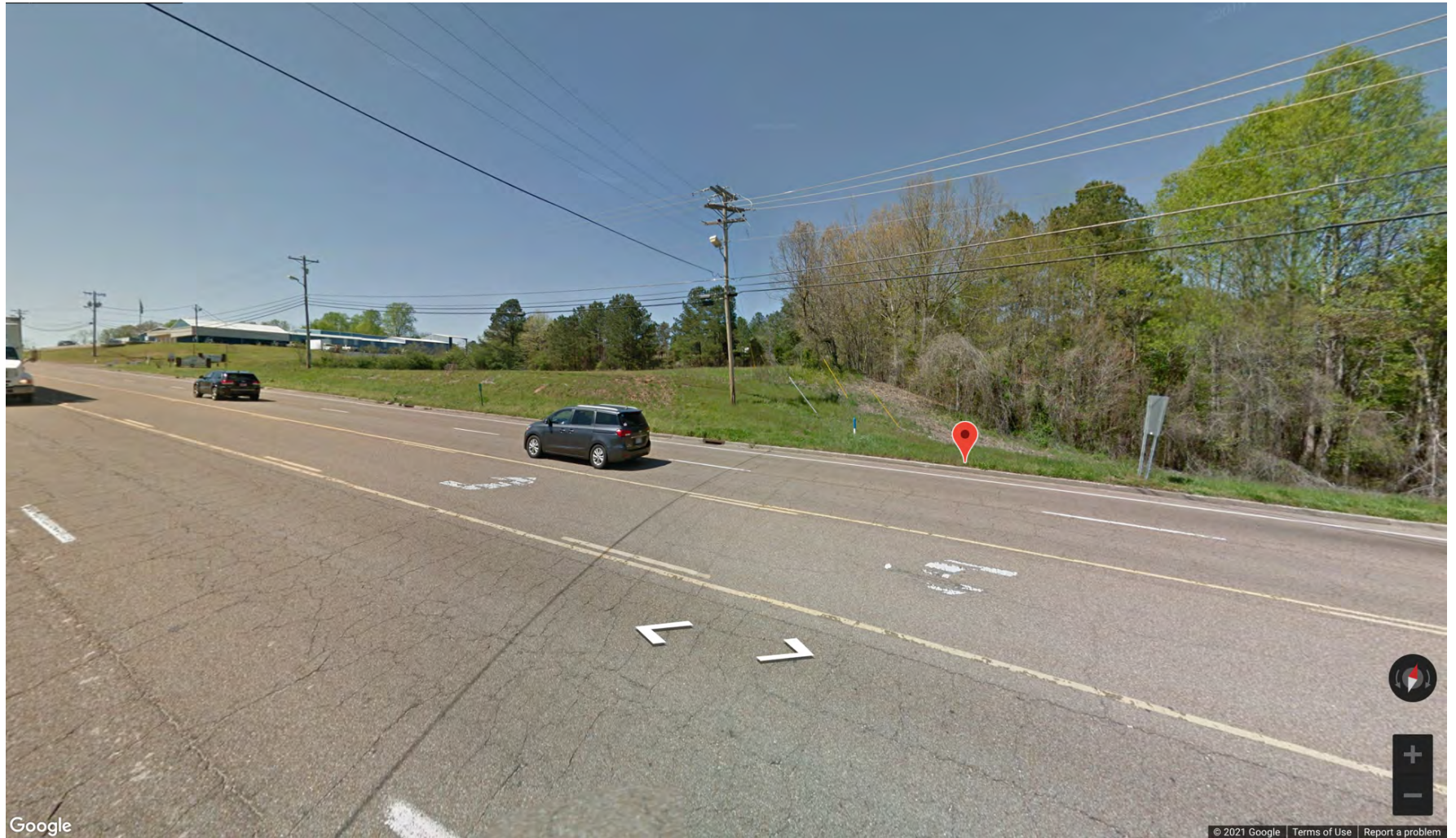
Camera 2, Solar Powered Safety Pole on Hwy 412 at Spur Dr.
