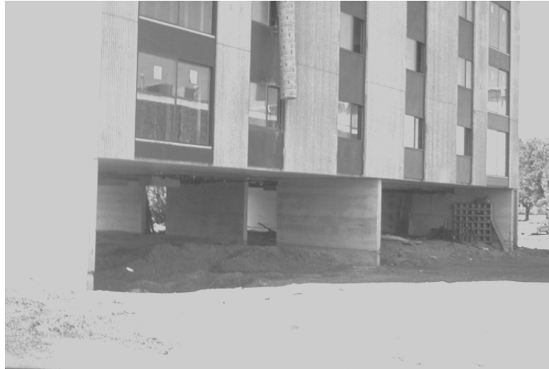
Figure 5-9: Building elevated on parallel stem walls.
